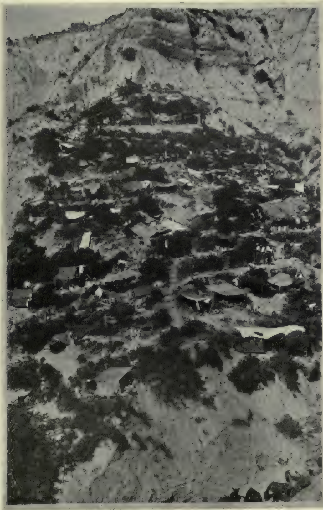
"DUGOUTS" CONSTRUCTED BY WELLINGTON MOUNTED RIFLES.
