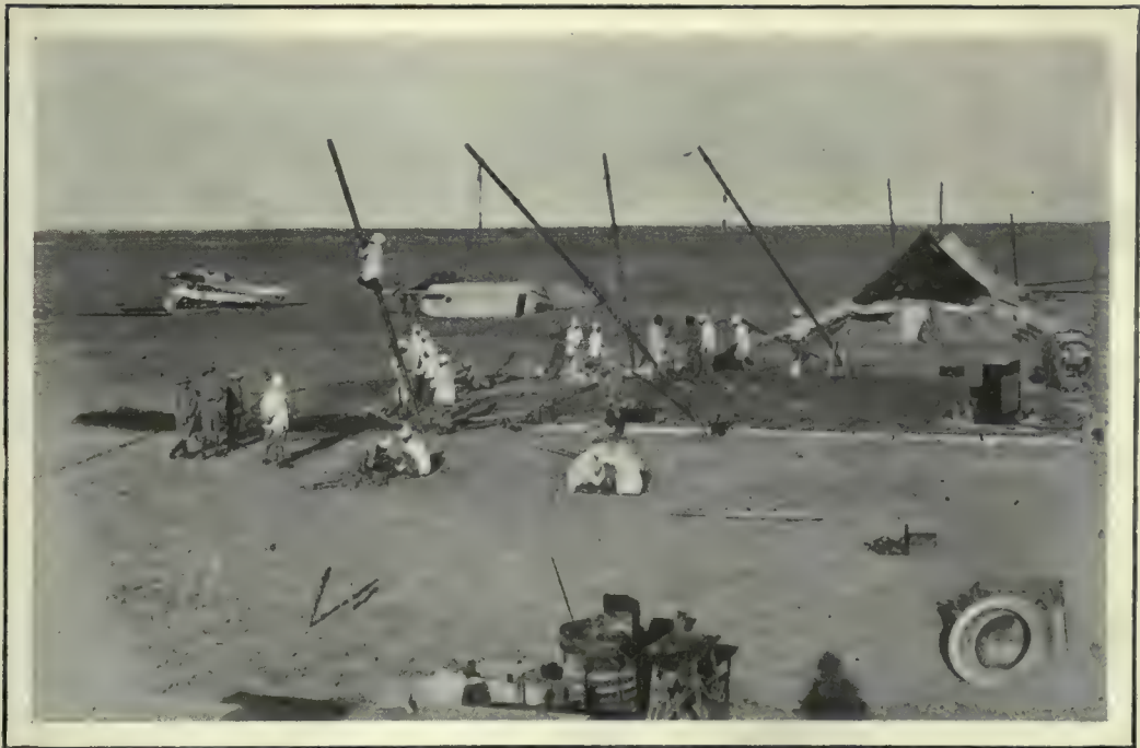
ERECTING PORTABLE CANVAS HANGARS IN THE DESERT.
