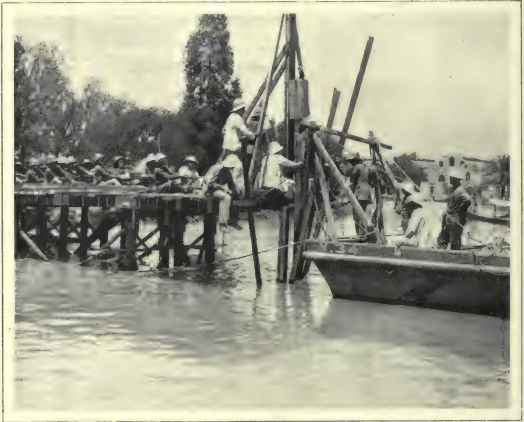
MAKING A NEW PIER AT BASRA : PILE-DRIVING BY MAN-POWER.
